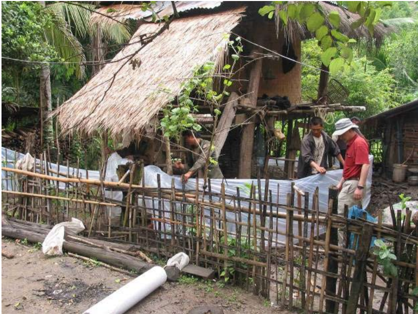
Fig 3. A grain store TBS being set up.
