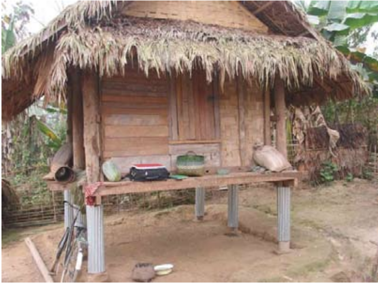
Fig 11. Grain store with support legs covered in corrugated metal to prevent rats gaining access to stored grain (unsure if effective).
